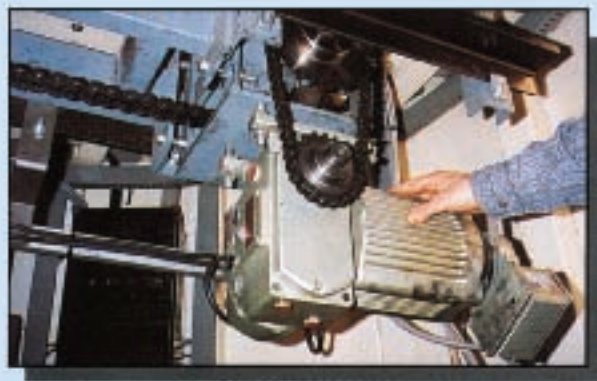
This page, clockwise from top left: cams to drive glass gates, positioned under platform; bridge locked in place with glass gate barriers; car controls for attendant; under car controller for bridge and gates; bridge motor unit located under platform; bridge extending to suspended floor, and bridge retracting
