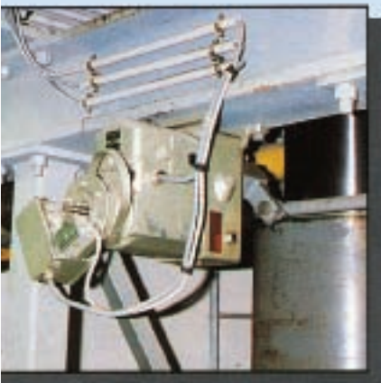
This page, clockwise from top left in machine room: motor unit for cylinder locking system; controller; tank with heat exchanger; rack and pinion stabilization units; hydraulic pump unit; safety sensors around cylinder and under car controls, and access shaft to plunger.
